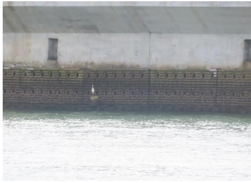
General View of Vertical Eco-shoreline
