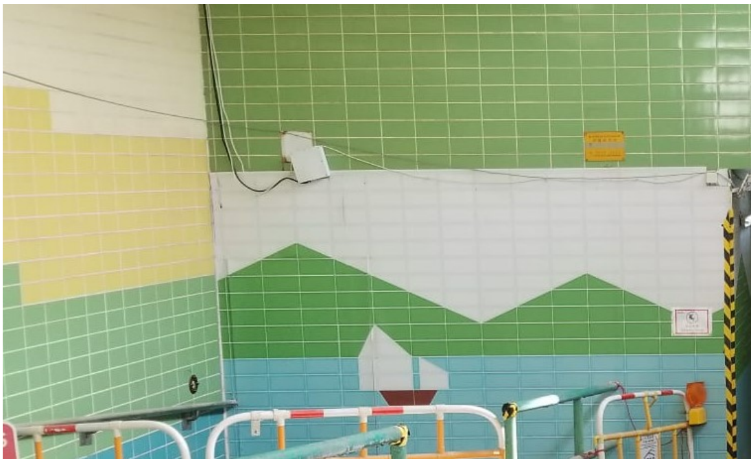
Photo 3 - Erection of site hoardings in unobtrusive colours
